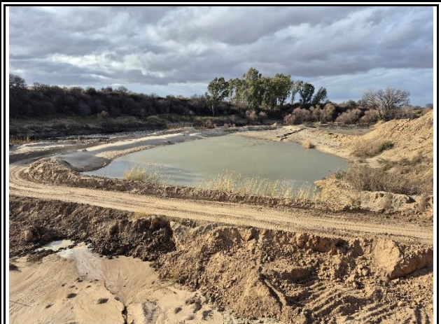
Settling ponds adjacent to the river where the berm was reinstated
